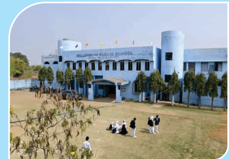
MILLENIUM PUBLIC SCHOOL HAZARIBAGH, JHARKHAND
